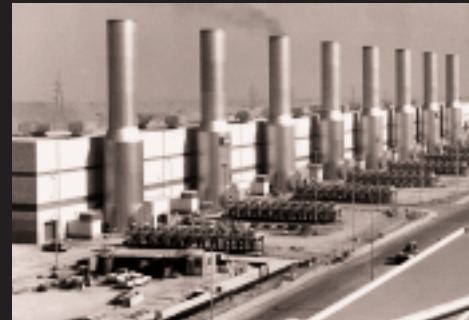
"Riad 8" gas turbine power station, Saudi Arabia
