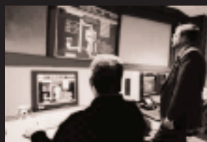
Control and instrumentation equipment for power station, ca. 1995
