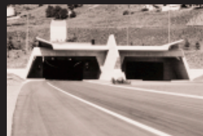
South entryway to Gotthard automotive tunnel with BBC control system, ca. 1982
